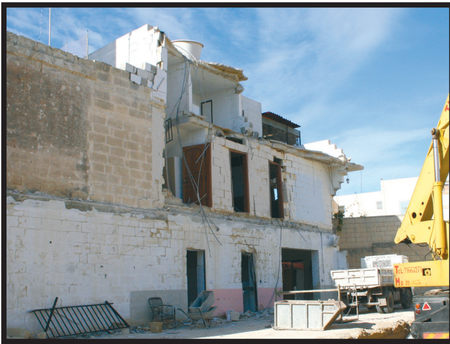
FOUR Naxxar families yesterday received €284,700 from the Housing Authority to be able to rebuild their houses that were destroyed by a fireworks explosion in a garage last March - see story page 3
